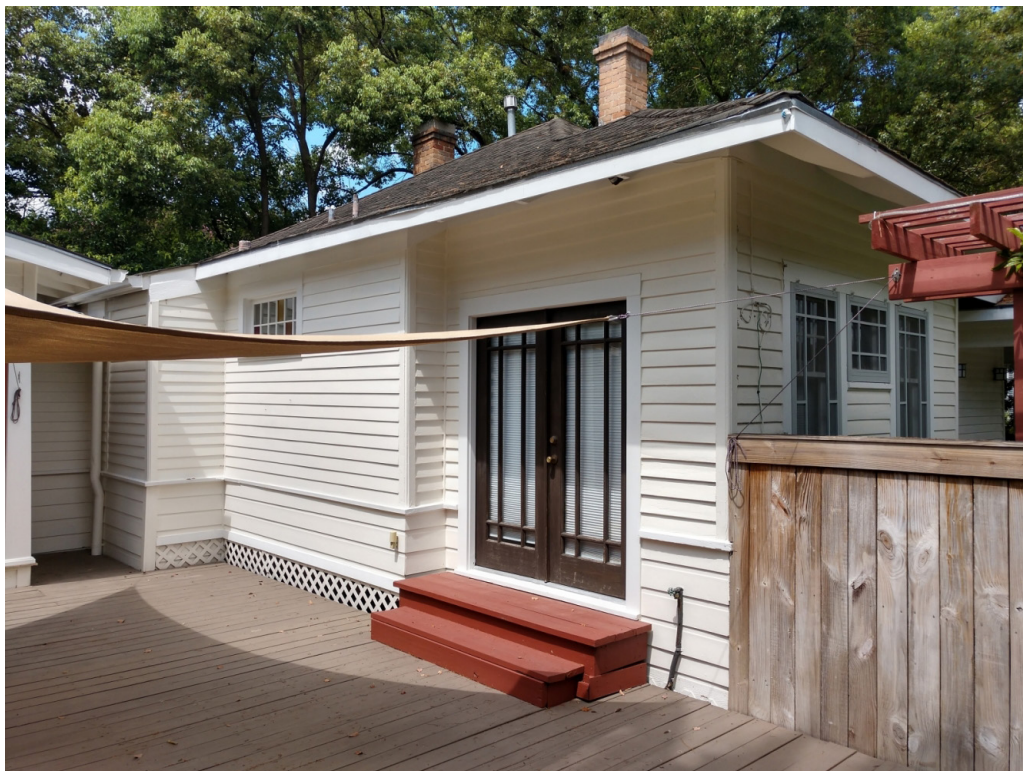
Southwest Corner- Existing West side, previously altered
