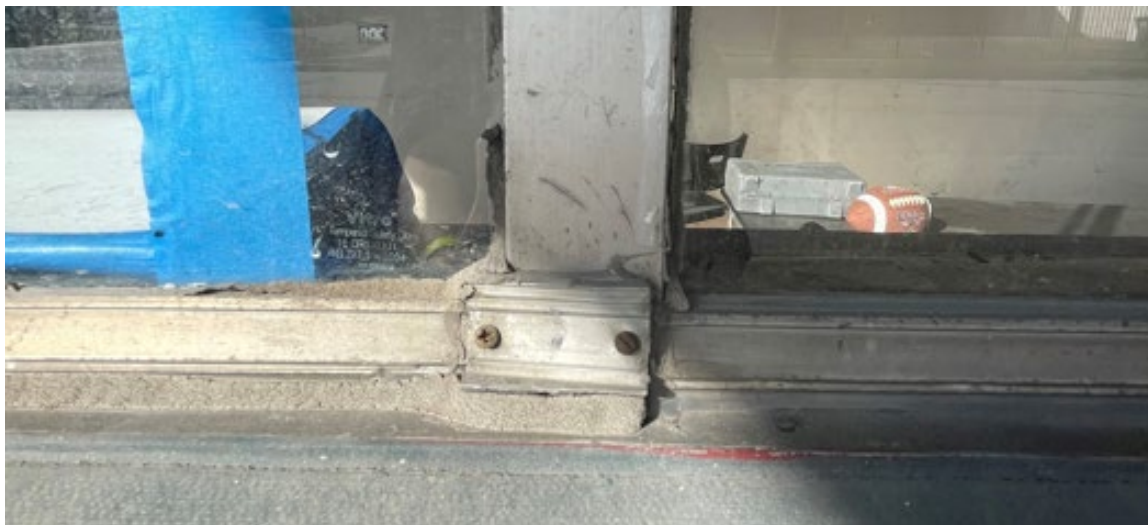
PROPOSED: NEW ALUMINUM WINDOWS, LARGER OPENING, LEVEL FAUX STONE VENEER TO MATCH ABOVE LEFT PHOTO
