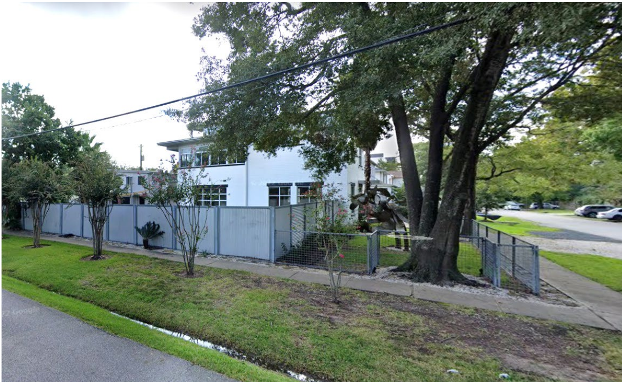
Figure 2- 448 Columbia St. across street from subject site – non-contributing
