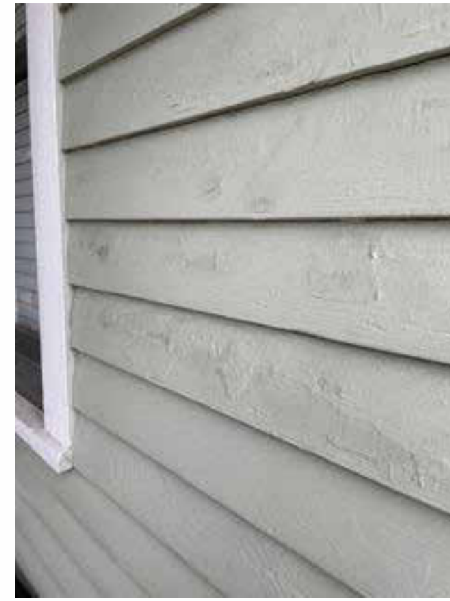
IMAGE INDICATES HISTORIC WOOD BEVEL SIDING WITH 4" REVEAL
