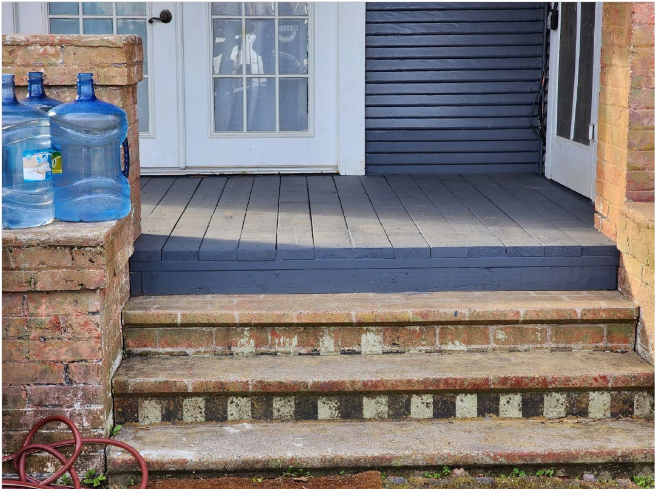
Figure 5 - Close up of new decking
