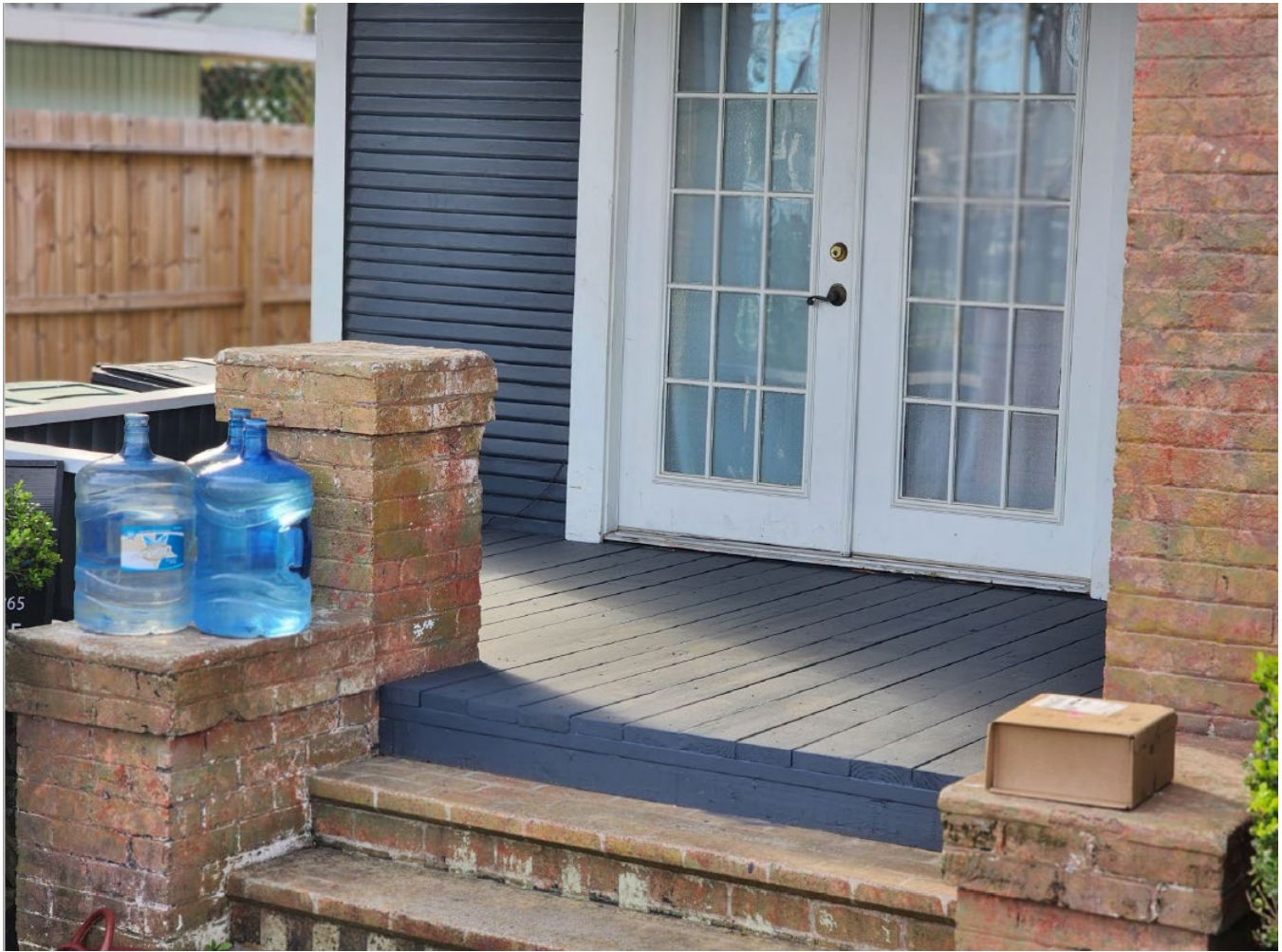
Figure 6 - Additional View Close Up of Deck
