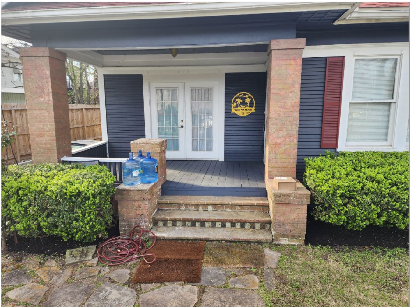
Figure 4 - View of porch floor after work completed
