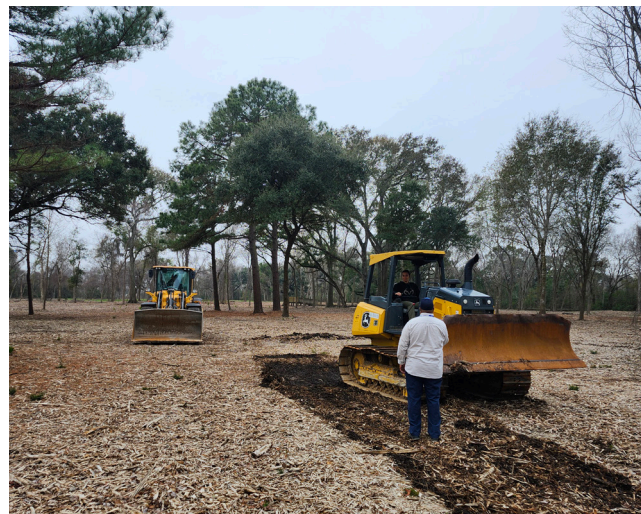
IMAGE: HPARD staff onsite in early phase restoration
