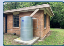
Rain cisterns help reduce the amount of water flowing during flood events. This decreases the amount of erosion and sediment in our bayous.
