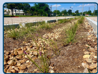
Native plants remove pollutants from stormwater runoff. This bioswale at Townwood Park acts as a filter, trapping sediment and chemicals during rain events.
