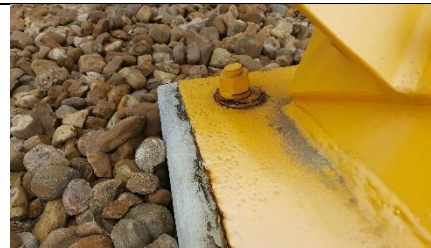
West of Pecos Artist: Rolf Westphal/ Ace Electric HAS Intercontinental Airport District B Completed Budget: $2,117.16
