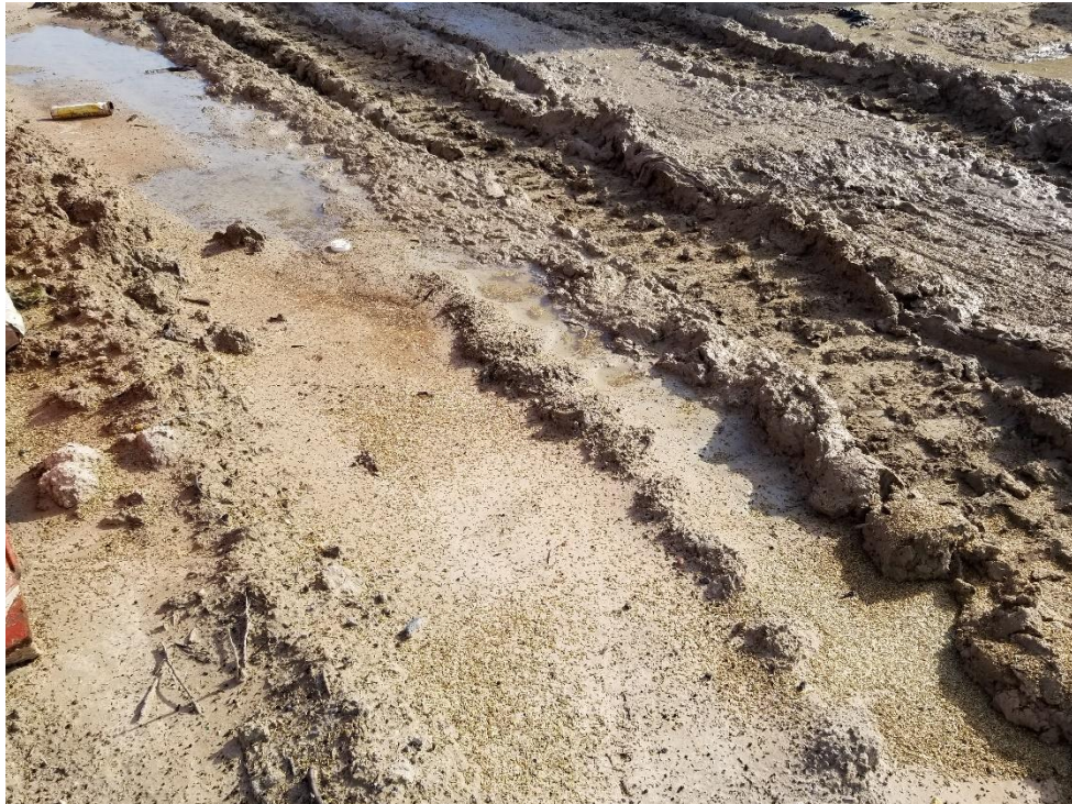
Grass Seed Has Been Spread Near Equipment and Storage Area
