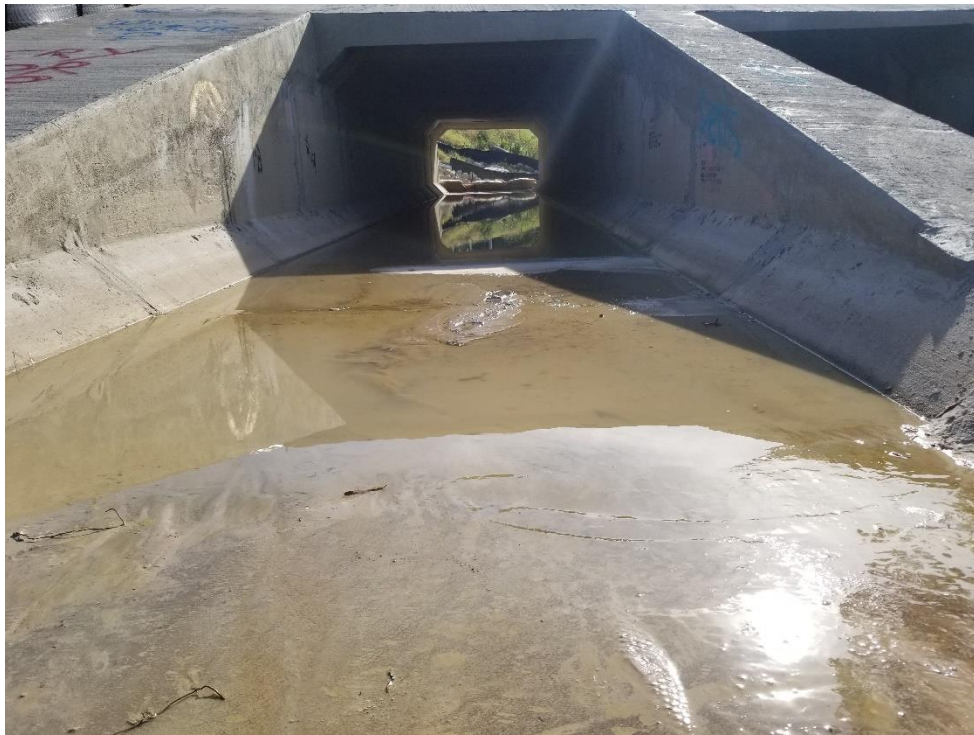
Light Sediment in Outfall Structure
