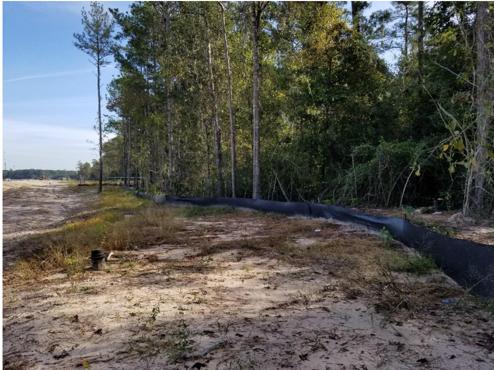
Well Maintained Silt Fence at Friarwood Drive
