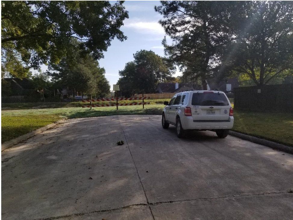
Curlex Blanket Stabilization at Creek Manor Drive Note: Street is clean
