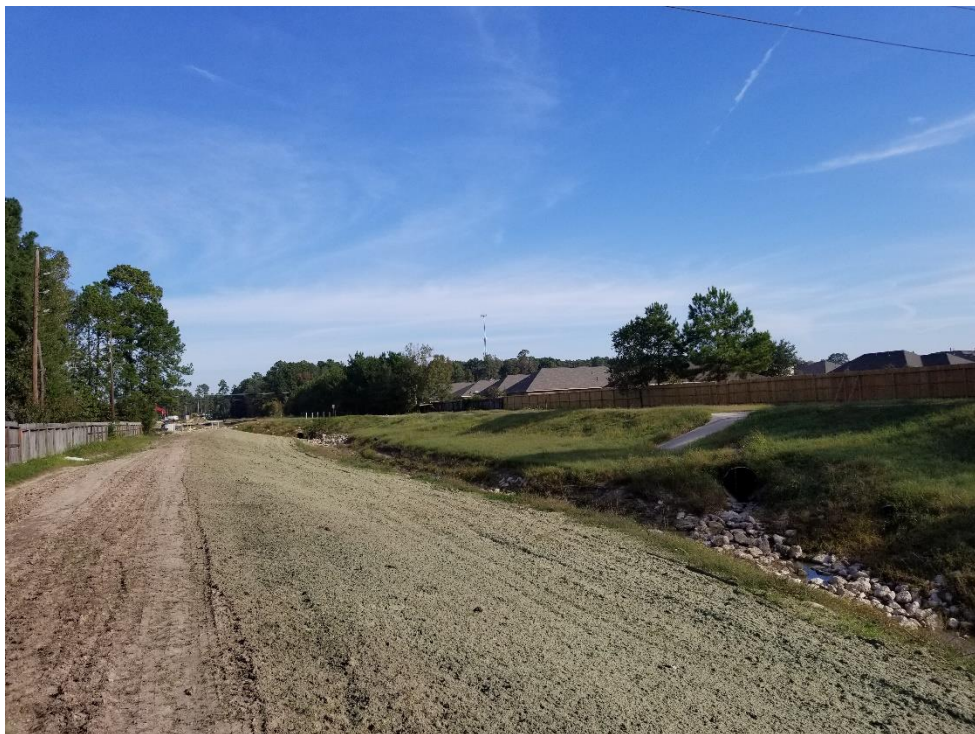
Hydromulch Applied on Slopes of Taylor Gulley
