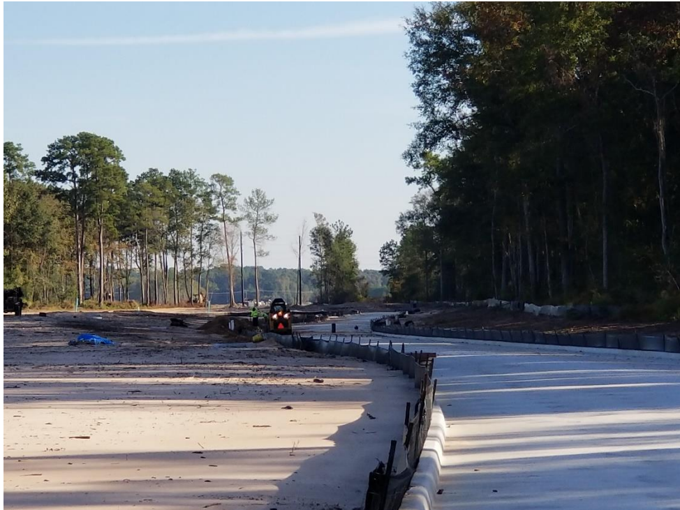
Construction Activity Taking Place near New Street in Development
