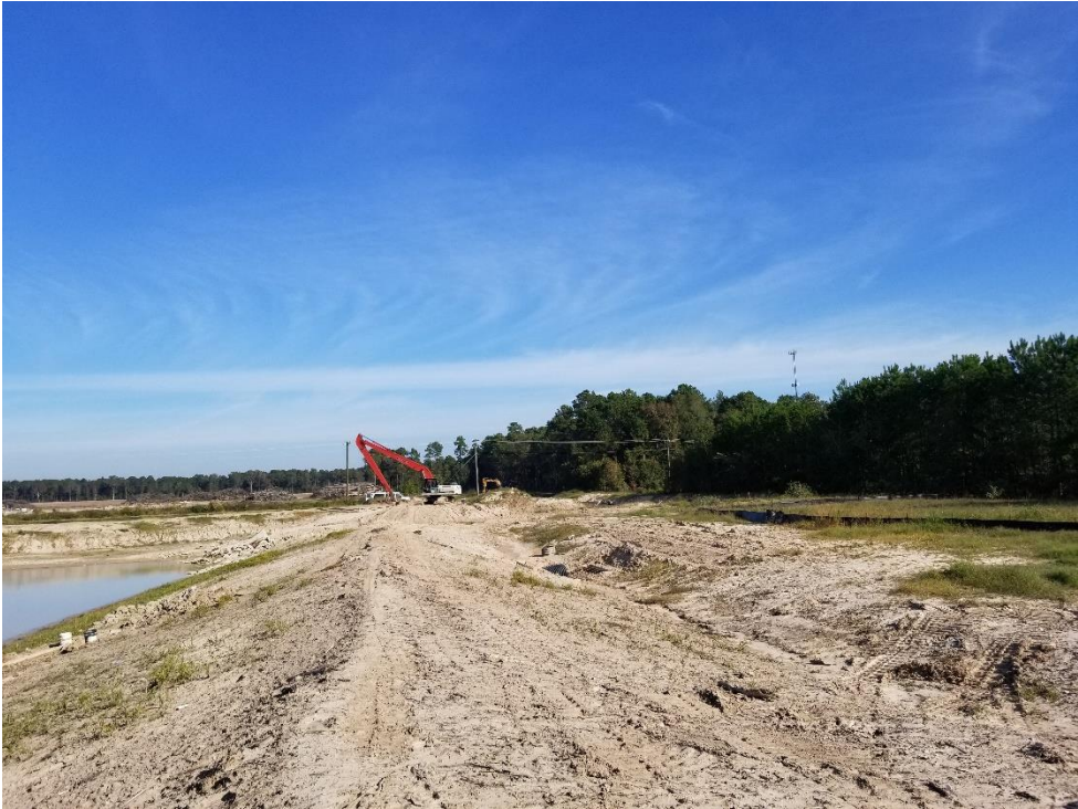
Construction Activity Taking Place Near Detention Pond #1
