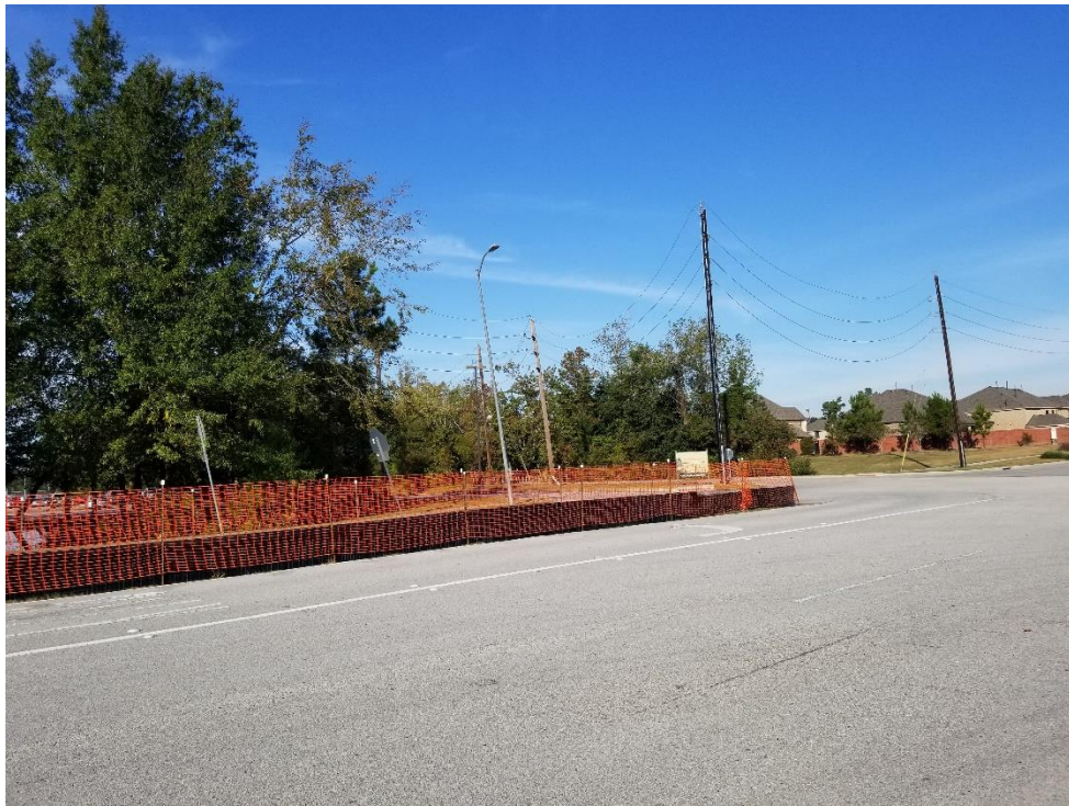
Median Protection on Woodland Hills Drive
