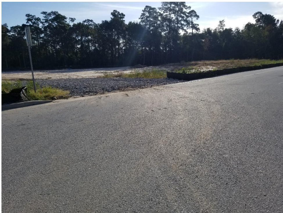
Construction Site Entrance on Woodland Hills Drive Note: Light sediment tracking
