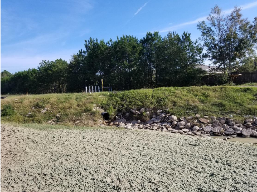
View of Montgomery County Ditch Outfall to Taylor Gulley
