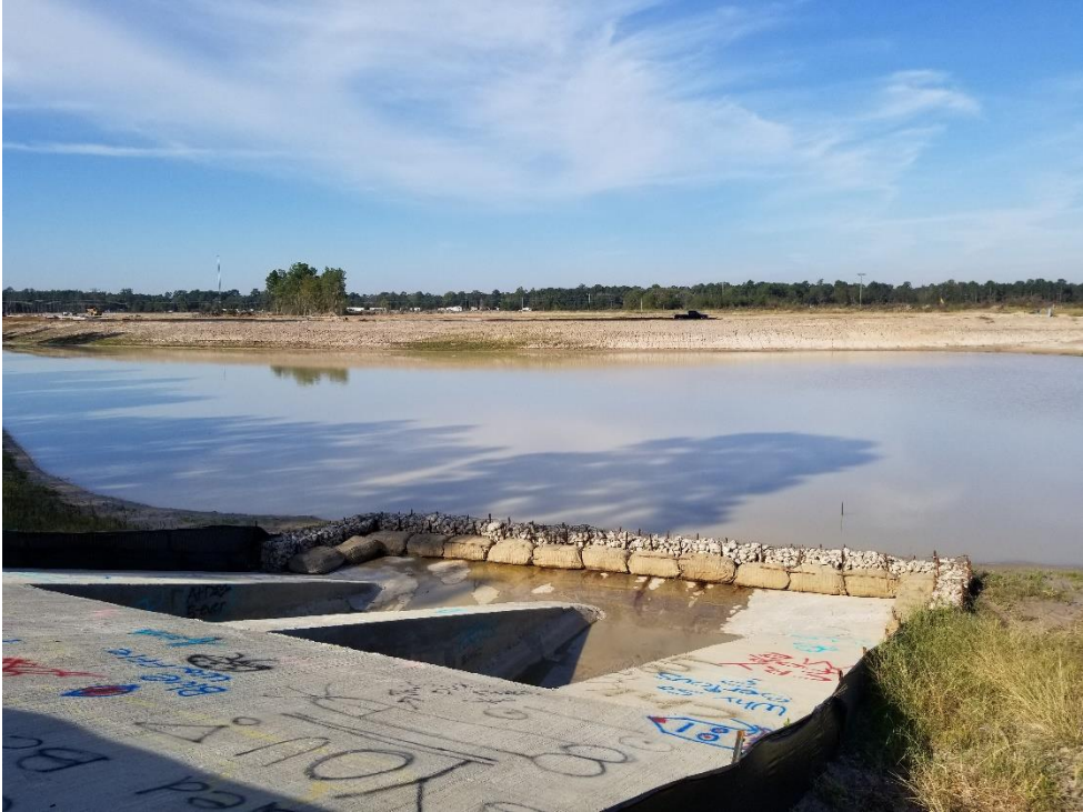
Hay Bales in Place at Outfall Structure
