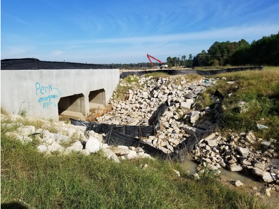
Outfall Structure from Detention Pond #1 to Taylor Gulley
