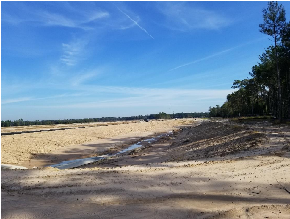
Detention Pond #2 Looking Northeast
