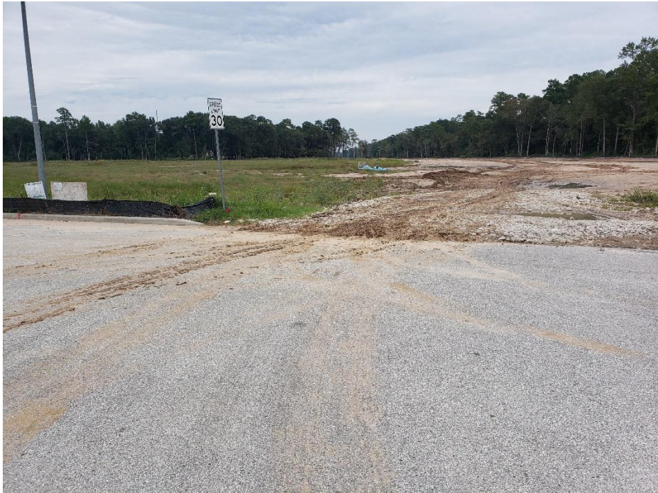
Construction Site Entrance on Woodlands Hills Drive
