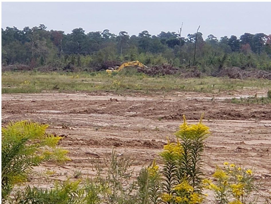
View Looking South from Webb Road Construction Entrance
