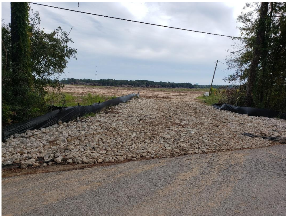
Construction Site Entrance on Webb Road Note: Light tracking
