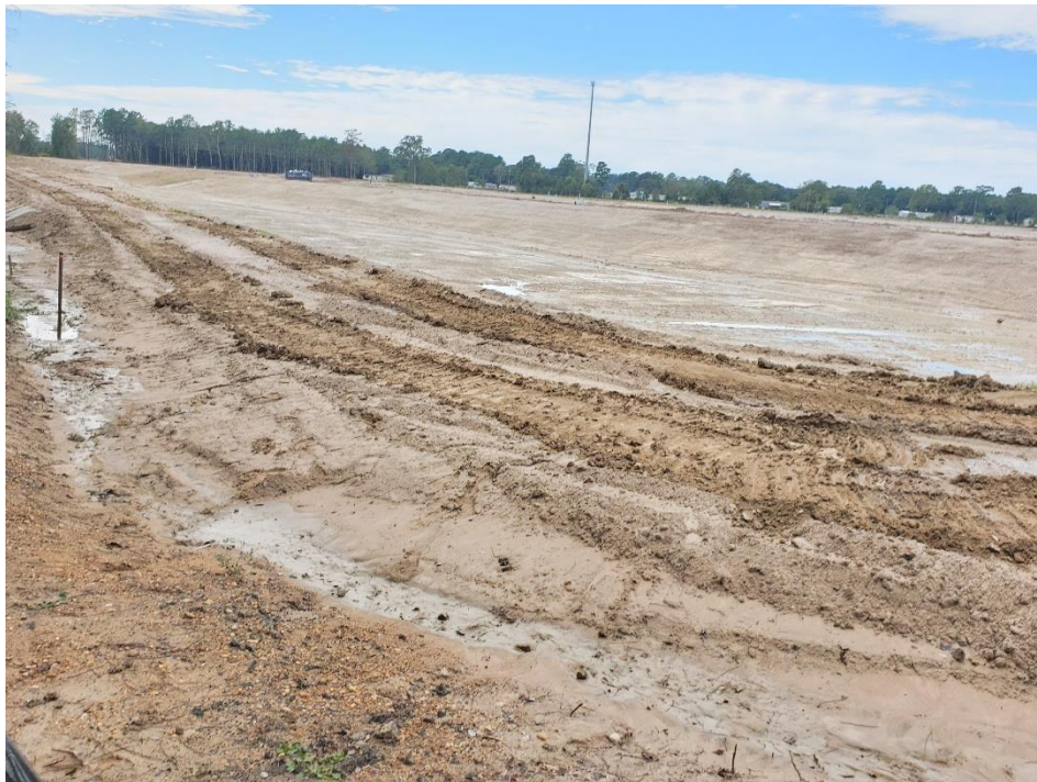
Second Detention Pond Under Construction Looking Northwest
