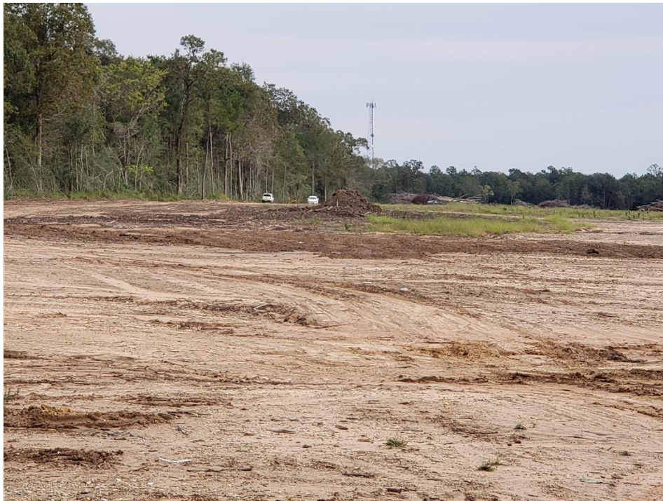
View Looking East from Webb Road Construction Entrance
