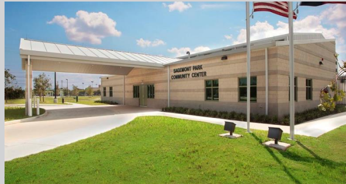
Sagemont Community Center & Park $3M
