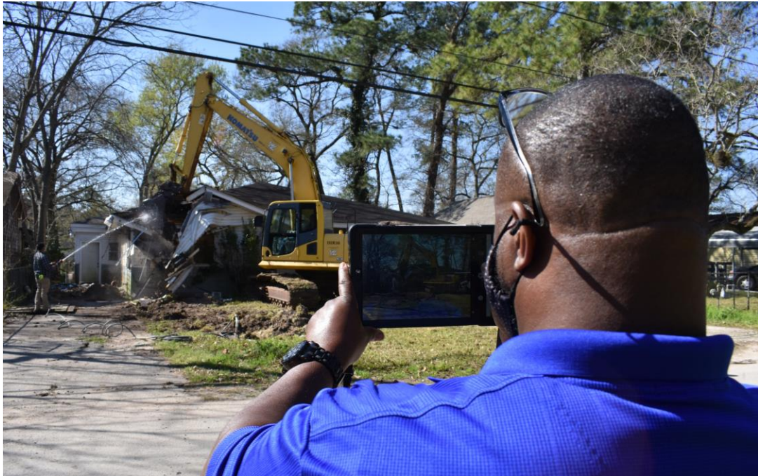
HCDD Inspector Leonard Pryce documenting the demolition.
