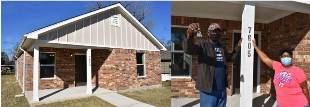
7605 South Hall, Houston, Texas 77028 (District B)
