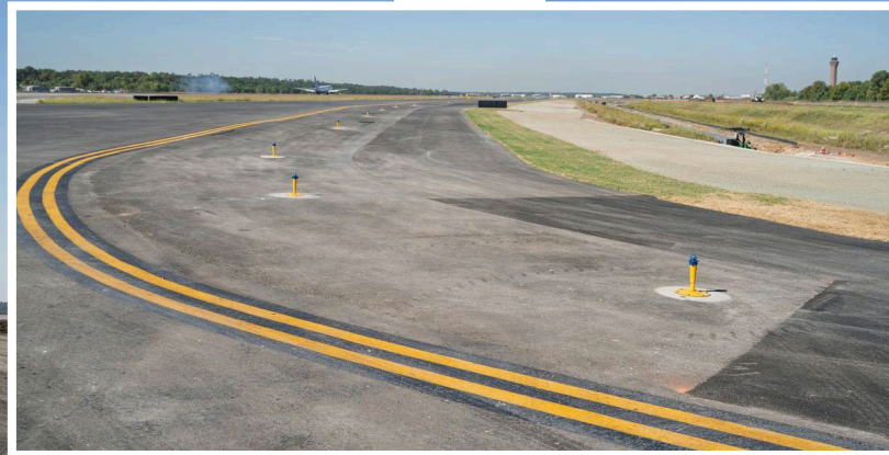
Taxiway SA: Asphalt Resurfacing Complete
