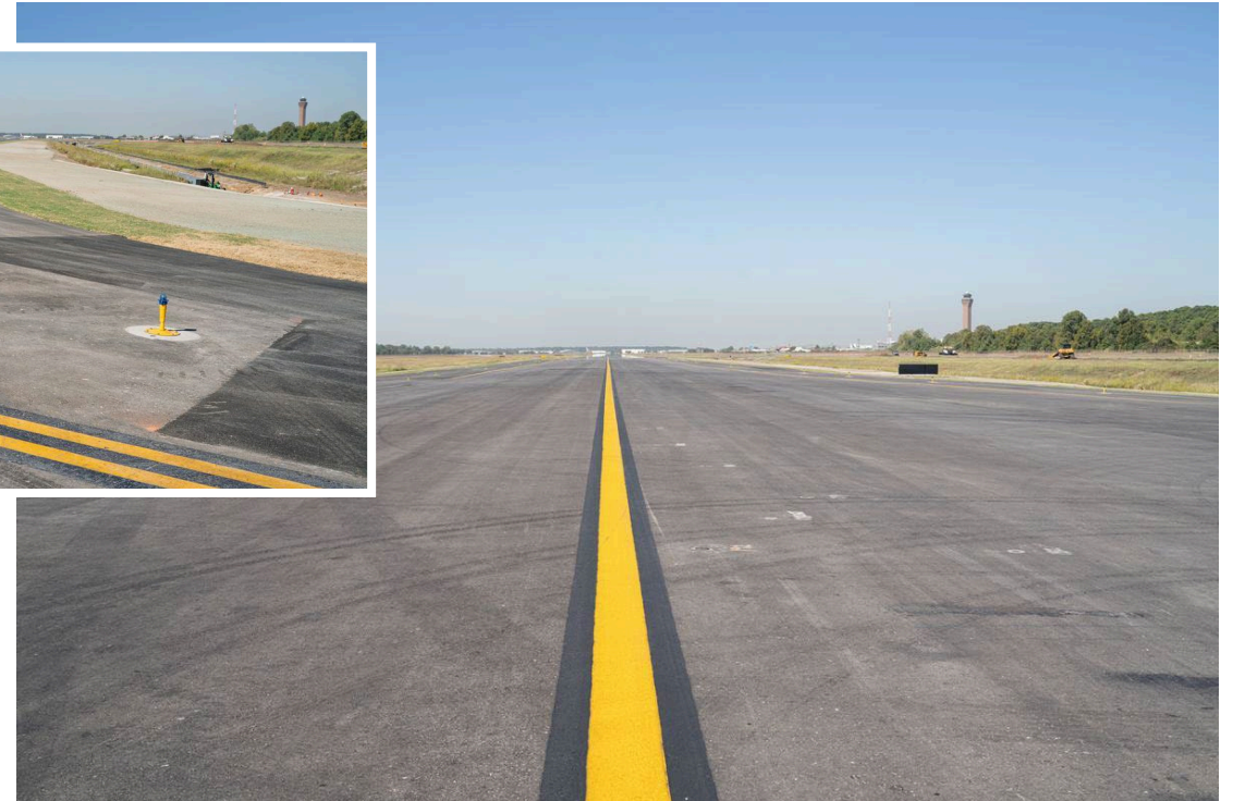
Taxiway SA: Asphalt Resurfacing Complete
