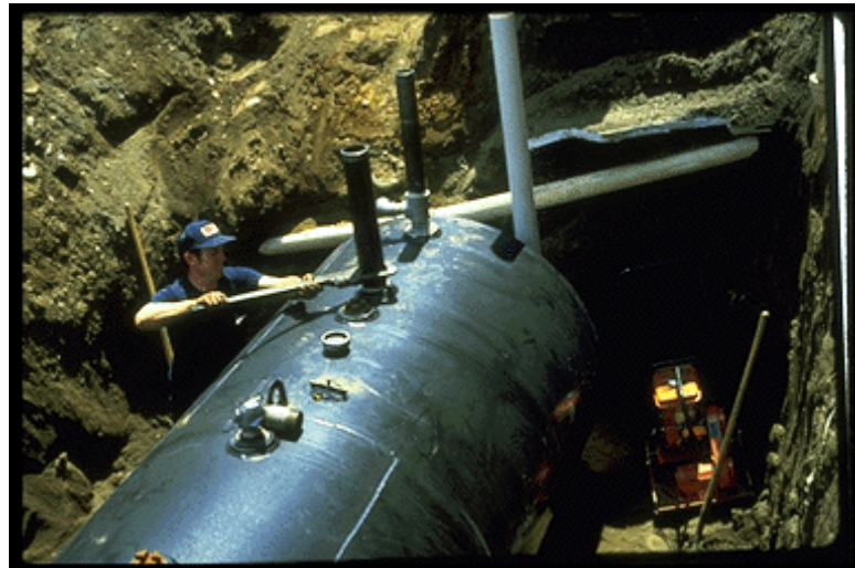
Underground Storage Tank being installed
