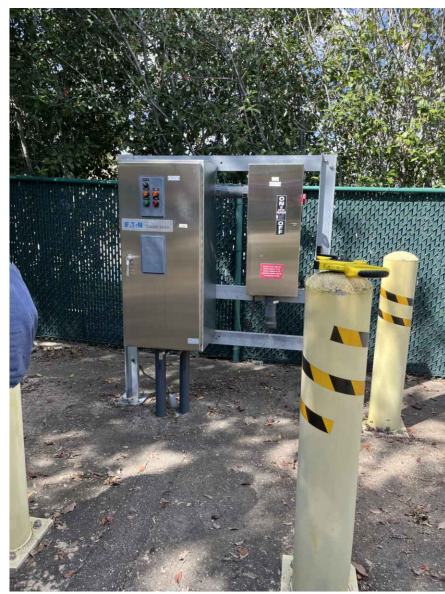
EXISTING GENERATOR PLUG AND DISCONNECT NTS
