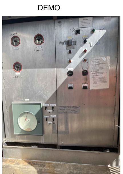
EXISTING LIFT STATION CONTROL PANEL
