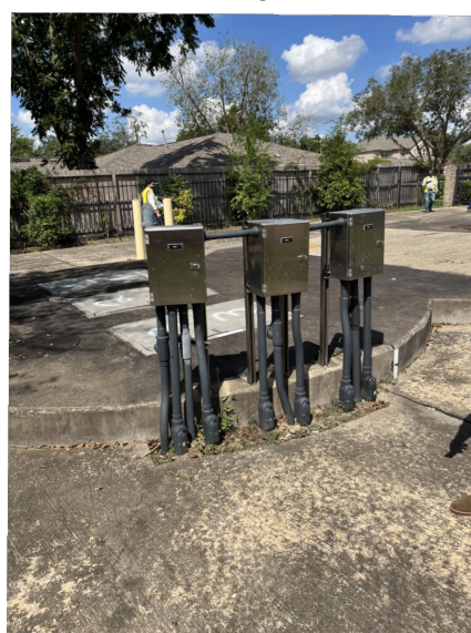
EXISTING LIFT STATION J-BOX (TYP OF 3) NTS
