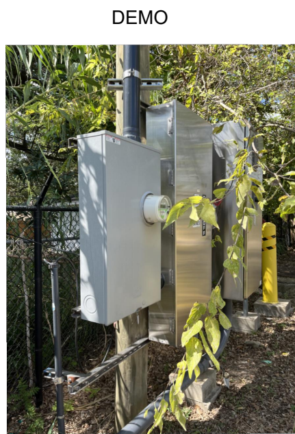
EXISTING LIFT STATION ELECTRIC SERVICE NTS
