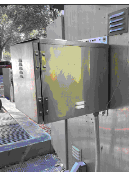
EXISTING LIFT STATION WIMAX CONTROL PANEL NTS
