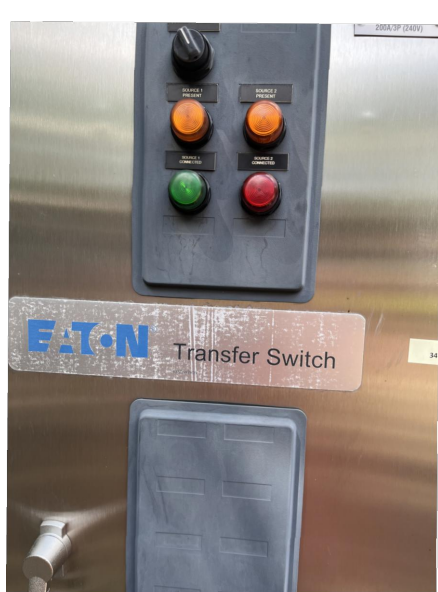
EXISTING AUTOMATIC TRANSFER SWITCH NTS
