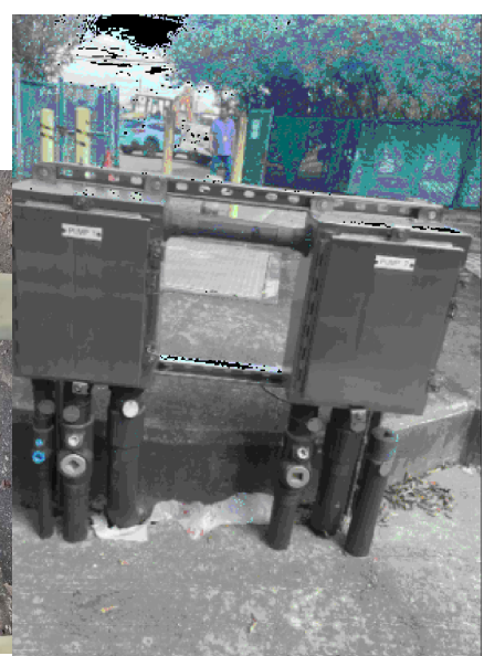
EXISTING LIFT STATION J-BOX (TYP OF 3) NTS
